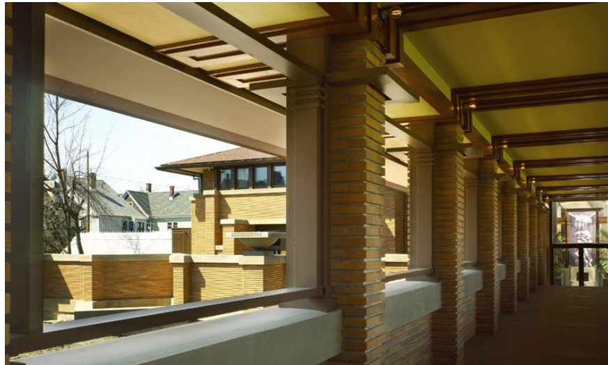
Reconstructed Pergola- Frank Lloyd Wright's Martin House- http://www.darwinmartinhouse.org/tour.cfm# .
