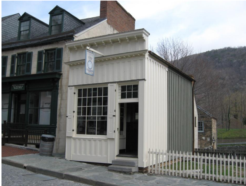
Reconstructed Alfred Burton Jewelry Store at Harper's Ferry National Historical Site-Photo taken by Alyssa Holland
